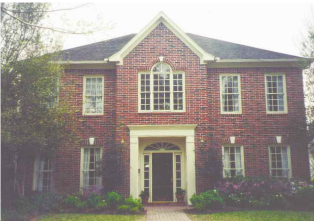
Figure 3: A row of vertical bricks centered with a keystone can also offer the complementary balance to the entablature over the door. Note the Palladian window placed directly above the main entrance or front door, with a keystone in the center arch.
