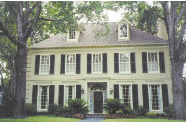
Figure 2: If the central doorway is framed with a decorative lintel or a classical entablature, the pairs of side windows should also have complementing lintels in either wood or stone. Dormers add a formality to the façade.
