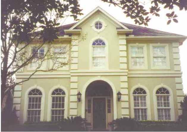
Figure 1: If the entrance over the doorway is arched, the windows on both sides of the door should also be arched. Note the round Roman window below the gable, detailed with four keystones.
